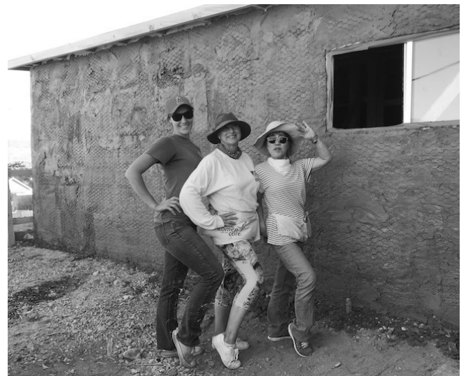
Hamming it up! The first coat of stucco is a rough "scratch coat" so that the smooth second coat sticks. Day groups from San Diego usually come to finish.
