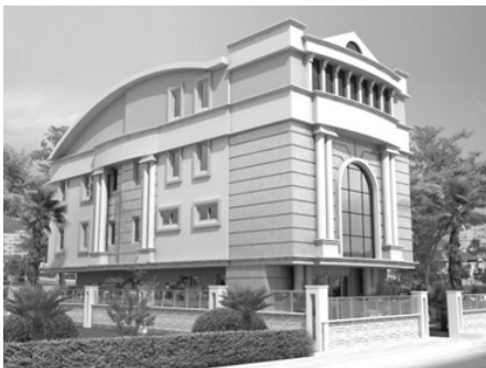
An artist’s rendering of the facility under construction for the Antalya Evangelical Church.
