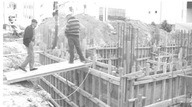
Photo from the church website: www.antalyaevangelicalchurch.com from last spring, showing foundations under construction.
