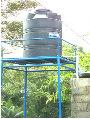
Water Tank Installed 2013
