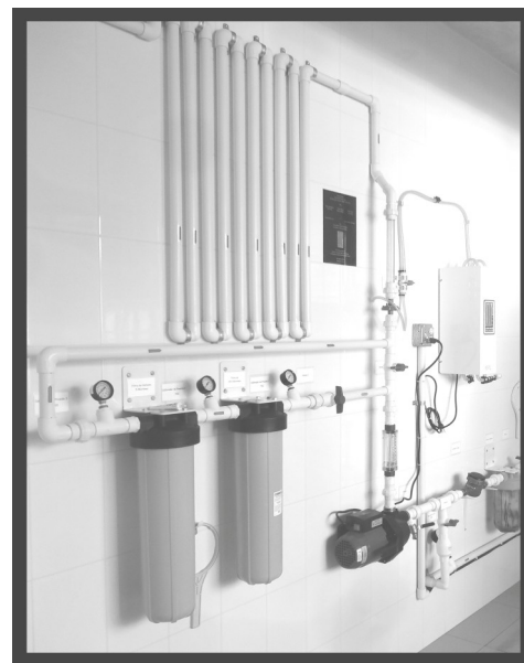
The water system installed and operating
